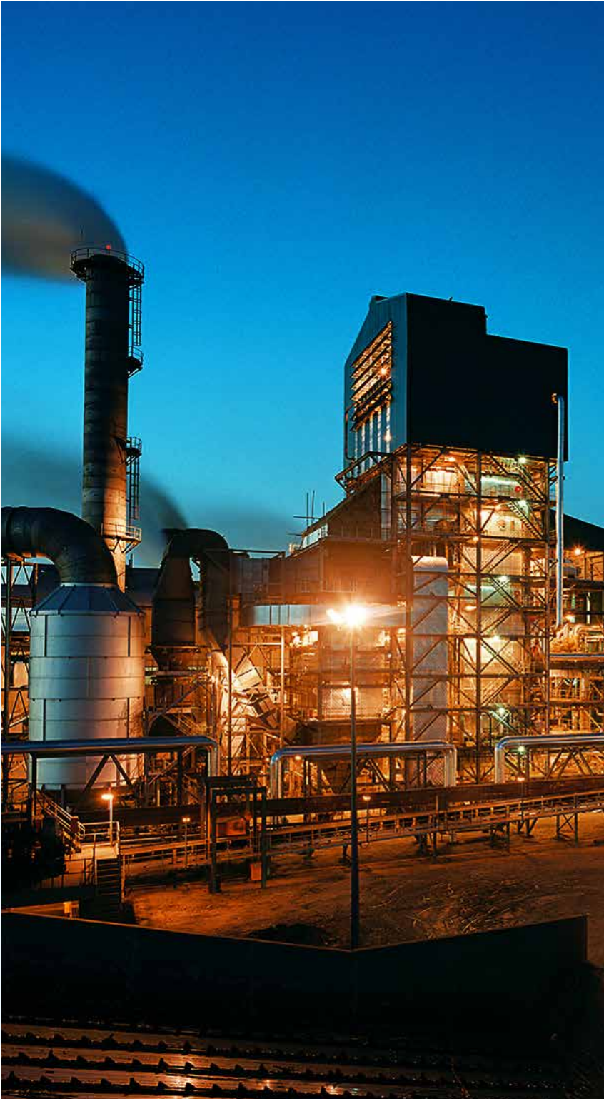
Night view of Boiler 6 at Nakambala Factory
