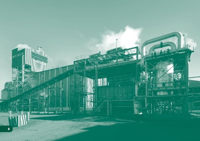
bagasse. Emission levels of sulphur dioxide and nitrogen oxides are low compared to conventional fossil fuels due to the characteristically low levels of sulphur and nitrogen contained in bagasse. The new boiler installed during the expansion project is fitted with a wet scrubber, which serves to remove almost all the particulate matter and gas from emissions into the atmosphere.
